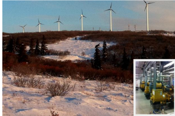
Figure 6: Unalakleet Wind Diesel System
