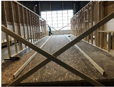
Figure 9: Double walls raised onto the floor.
