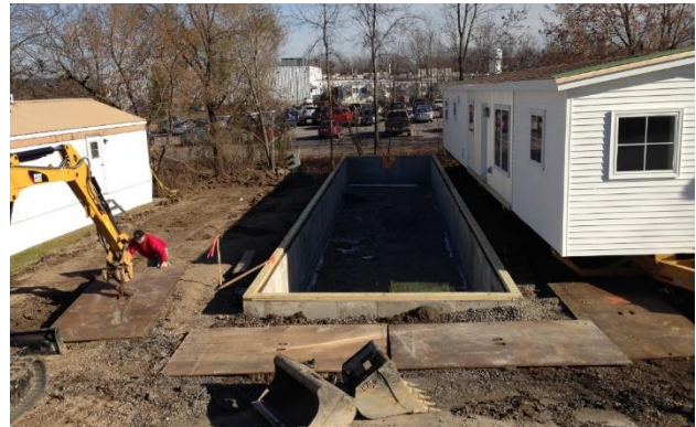
Figure 3: ZEM home being installed on a crawl space.
