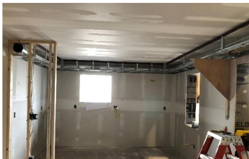
Figure 12: Installation of HVAC soffit and interior partitions.
