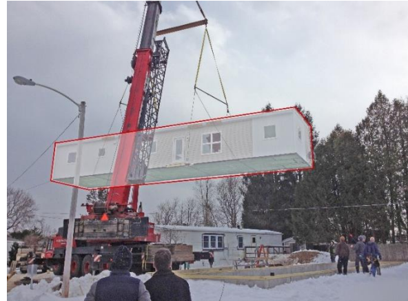
Figure 21: Setting of a ZEM MMH replacement onto its foundation.
