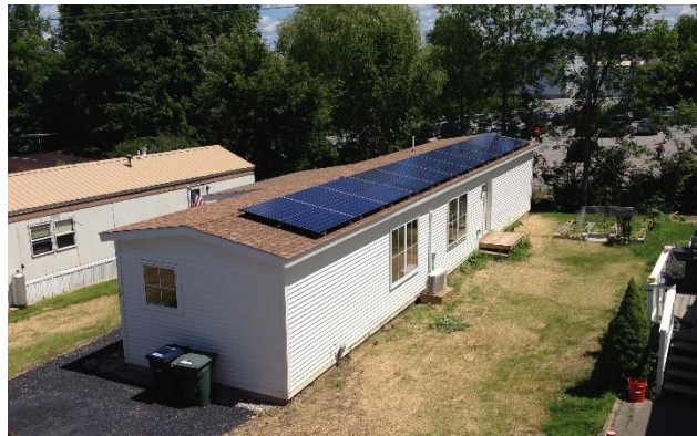
Figure 5: ZEM low-pitch roof in a MMH replacement project
