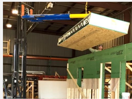
Figure 10: Crane lifting roof onto walls.
